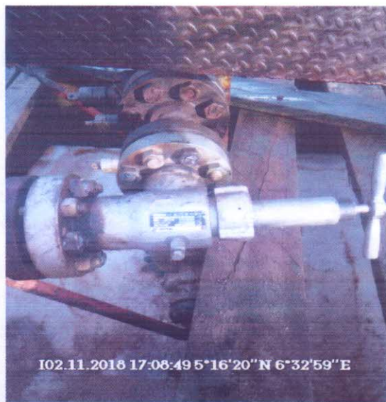
Fig D: After replacement and repair.
